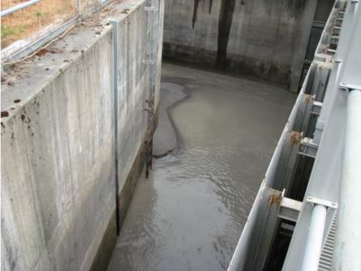
Figure 22 Sediment accumulation in the channel and the third gate at the channel edge.
