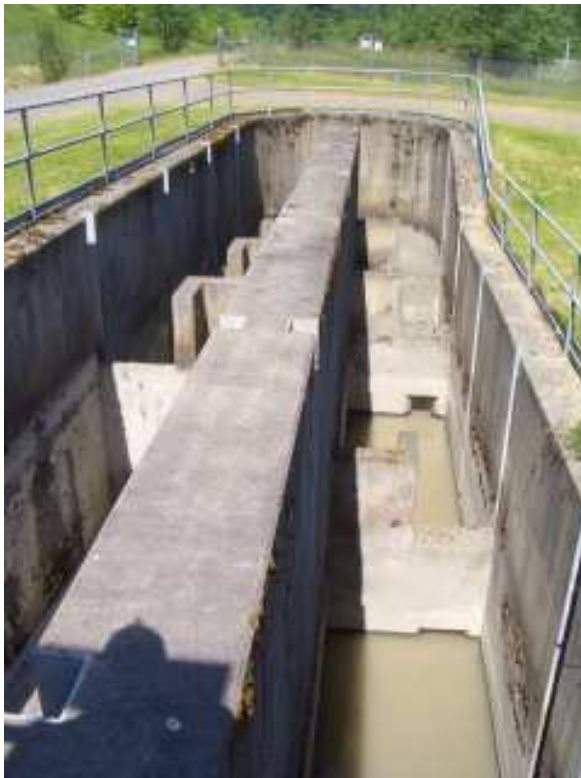
Figure 3 Components of the Fish Collection Facility (FCF). Counter-clockwise from top: the fish barrier dam; fish ladder; and terminal trap.
