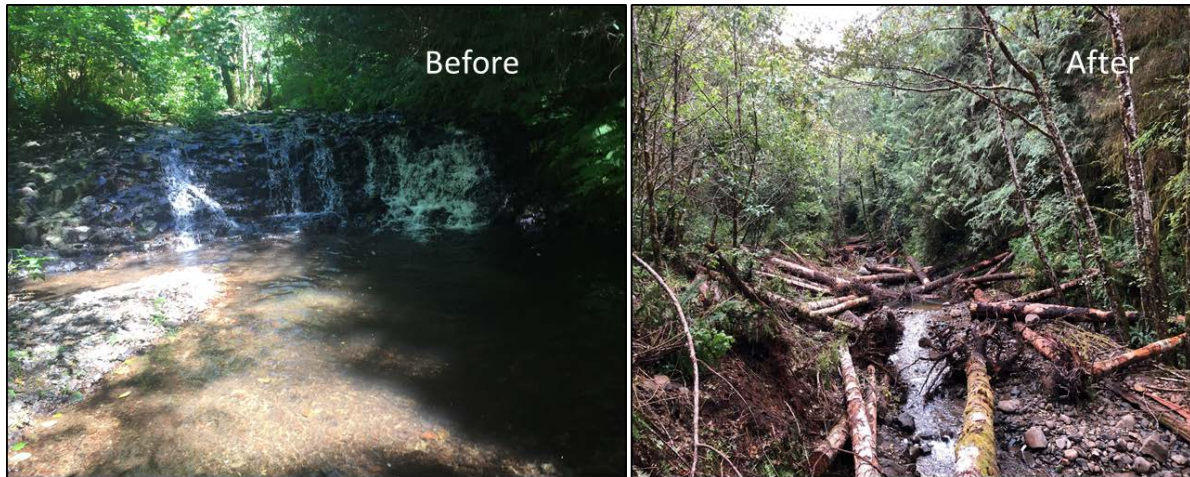
Figure 11. Pictures of Sarah Creek before and after project implementation. Streambed aggradation and LWD placement effectively removed a barrier that opened-up nearly one mile of habitat to anadromous salmonids.
