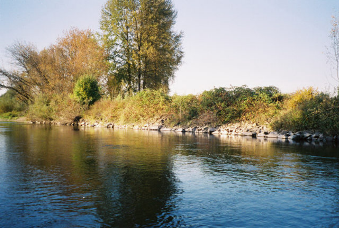
Figure 4. 6. Riprap bank protecting the airstrip on the lower mainstem East Fork Lewis River. Photo taken September 2004.
