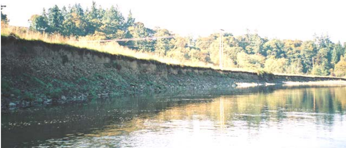
Figure 4. 48. Photo of eroding streambank in reach 8A (RM 9.7).
