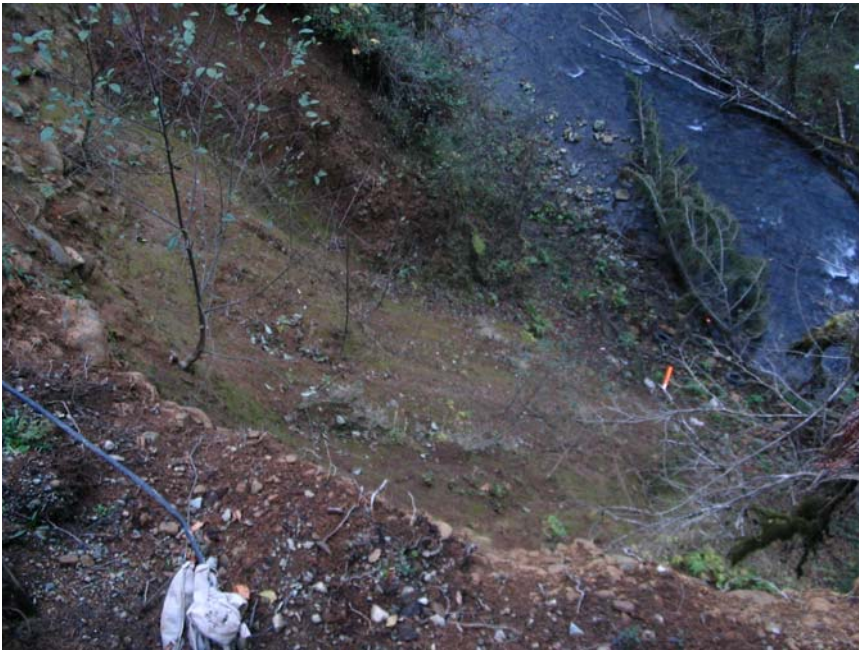
Figure 4. 23. Landslide from road failure (Dole Valley Road) directly entering Rock Creek.
