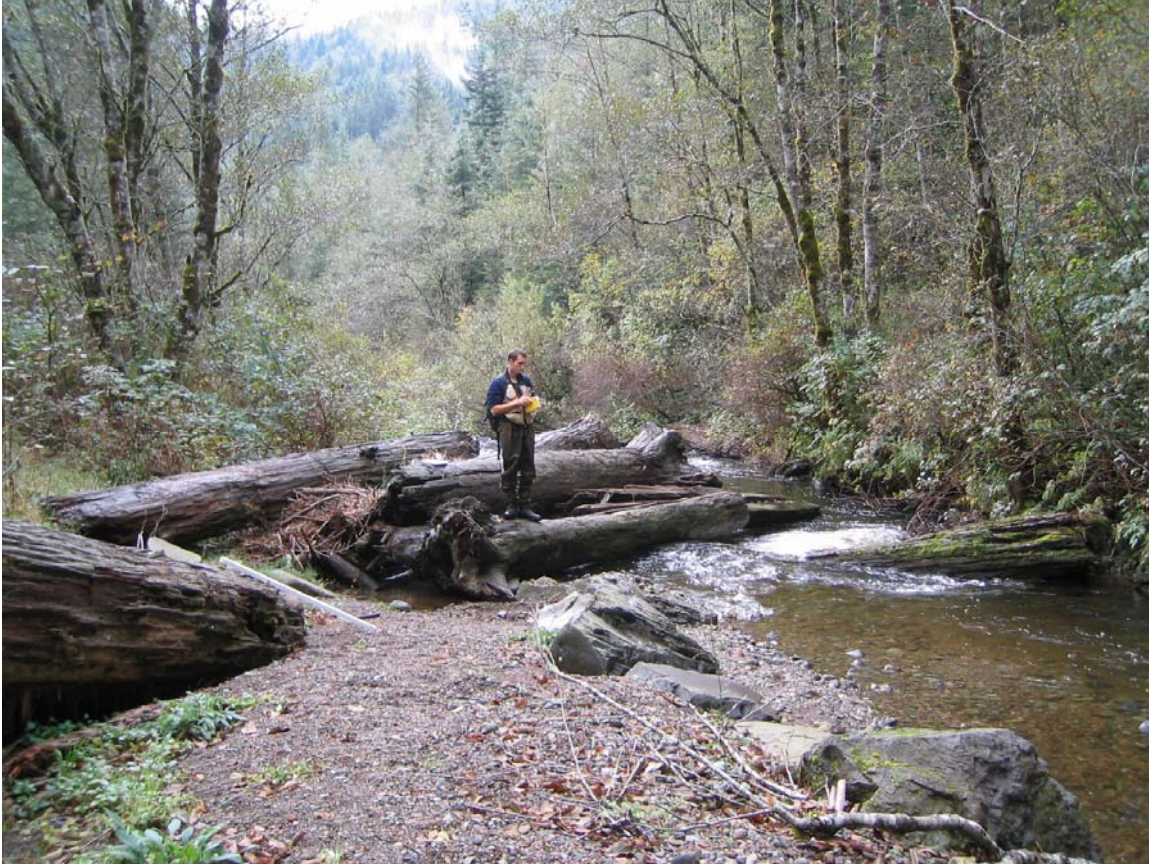
Figure 4. 121. Photo of stream restoration activity in lower Slide Creek (view looking downstream). Note buildup of cobbles and gravels upstream of engineered jam and formation of pools both above and below the jam. The de-commissioned road is approximately 5m off to the left of the picture.
