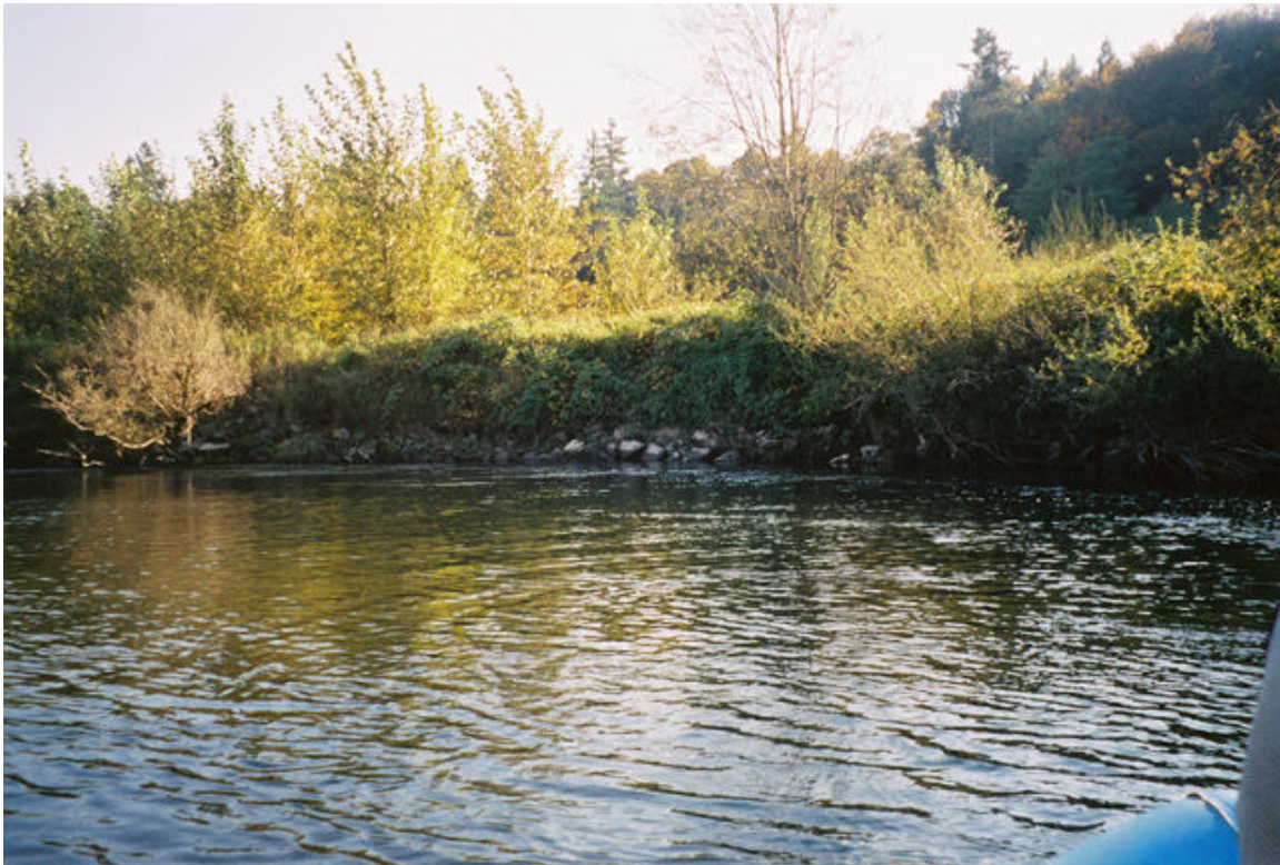
Figure 4. 31. Rip-rap bank on south bank at RM 6.8.
