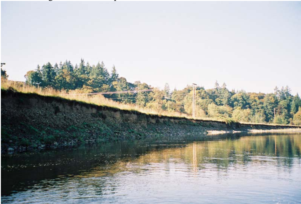
Figure 4. 27. Erosion of alluvial terrace at downstream end of Reach 8A (RM 9.7). This property has been acquired by the Columbia Land Trust and offers good restoration potential.
