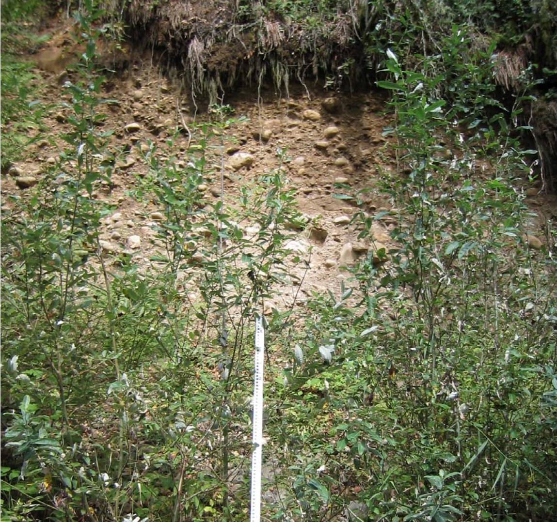
Figure 4. 91. Actively eroding bank of Lower Rock Creek contributing fines, gravel and cobble to the stream.
