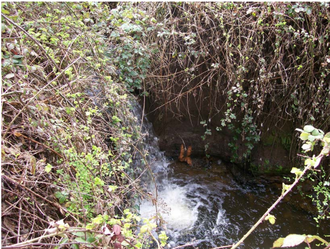
Figure 10. Waterfall at headcut nickpoint locate approximately 100 feet upstream of Padden Parkway.
