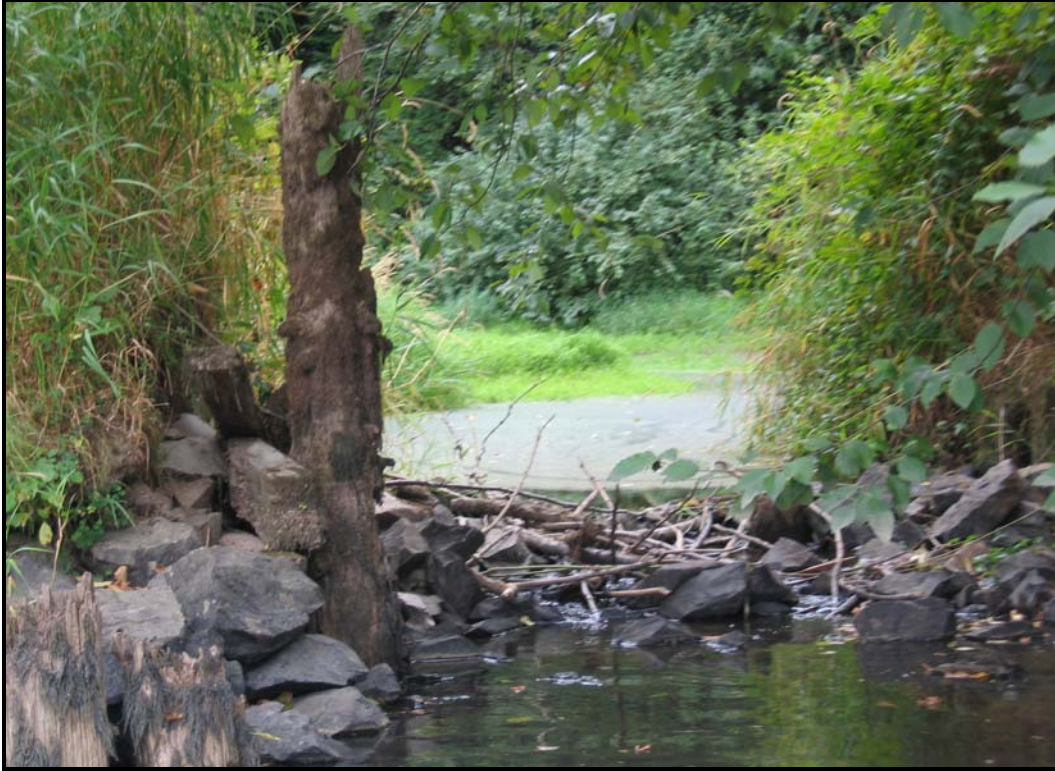
Image looking at Hill Creek outlet through historical railroad embankment near RM 24.0
