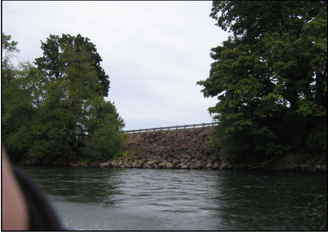
Image looking at left bank near RM 26.3, just upstream from previous photo.
