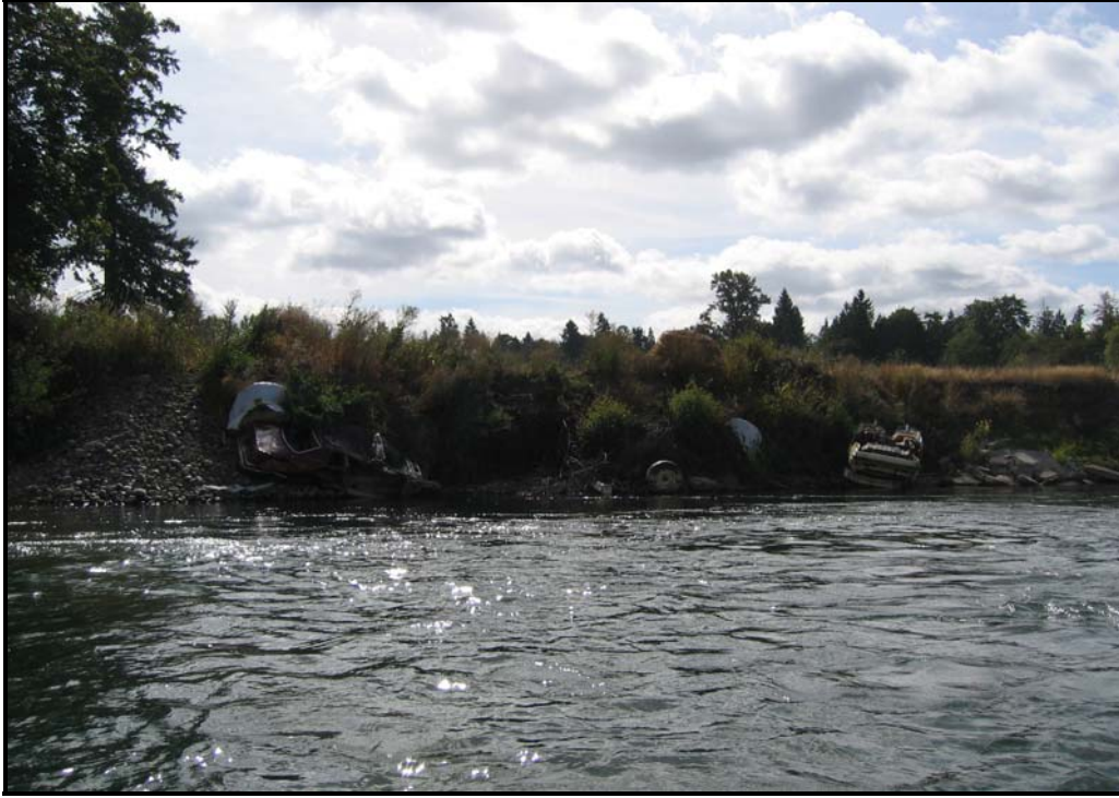
Looking towards left bank with car revetments protecting agricultural land near RM 32.5
