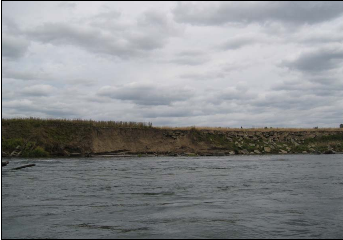
Image looking at left bank near RM 26.0
