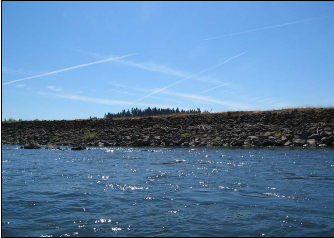
Image looking towards left bank at Kirkendoll Levee near RM 37.5
