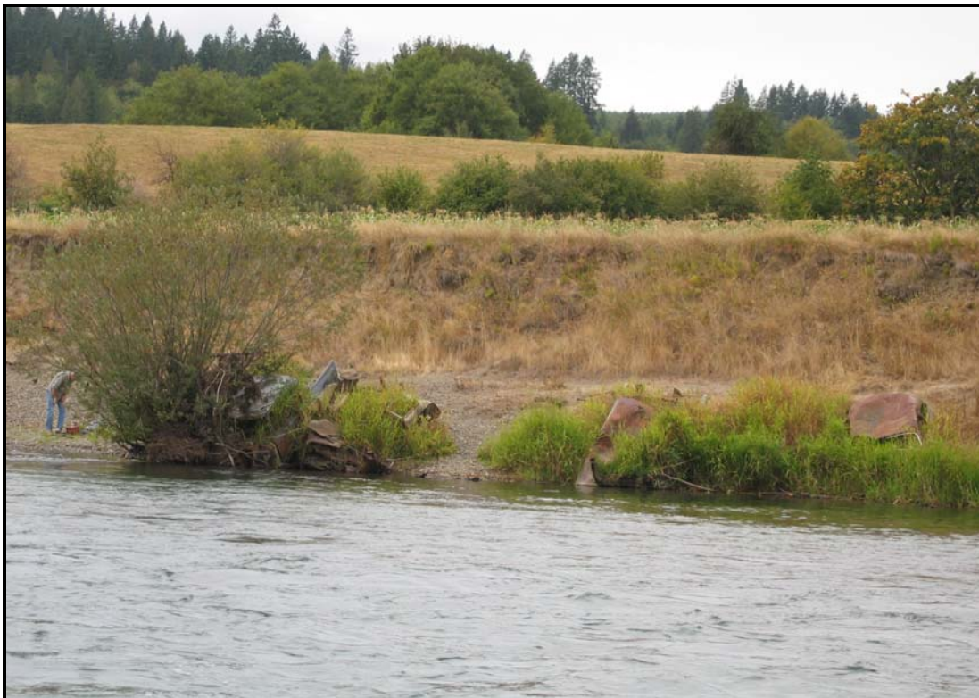
Image looking toward right bank at car “revetment” near RM 25.2.
