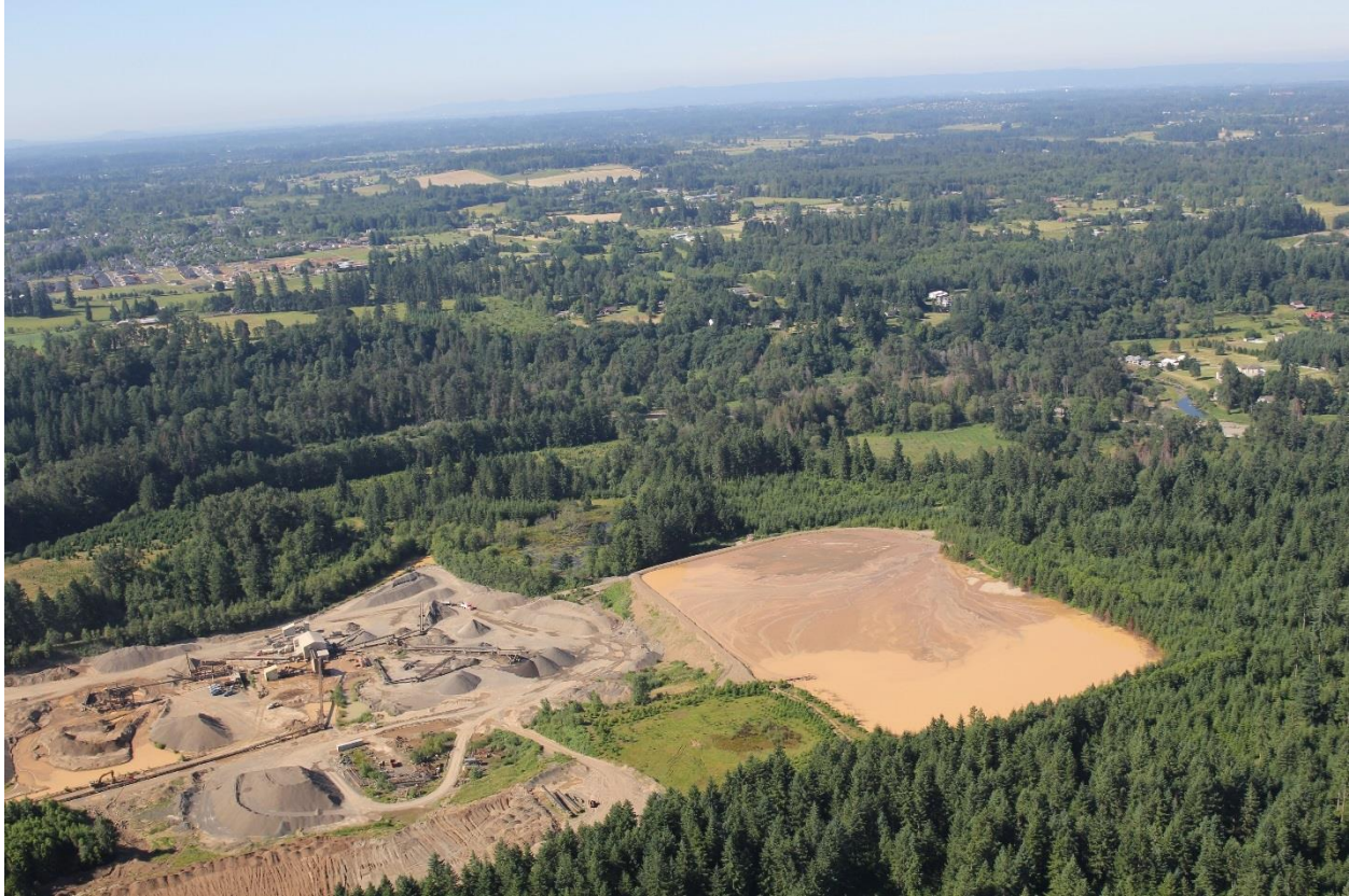
Figure 27. Lewisville Pit perched directly above the EFLR floodplain. Photo taken June 13, 2019 looking South.
