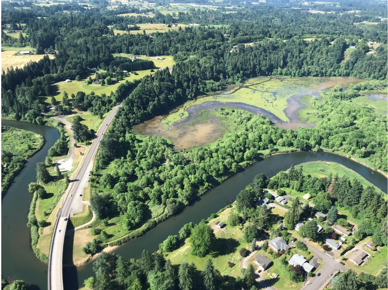
Figure 31. Photograph of the La Center bridge crossing the East Fork Lewis River, oriented south. Image taken in 2019.
