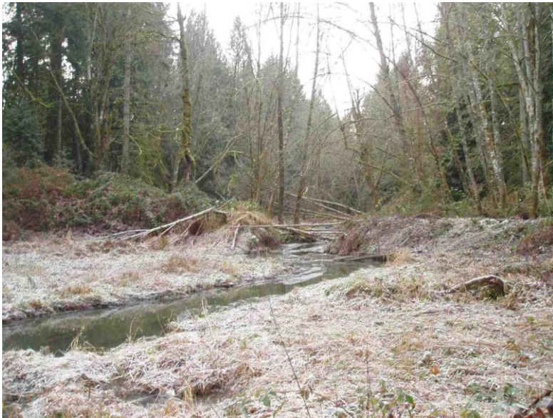
Figure 39. Remnant floodplain fill spanning the floodplain near RM 7.3. The creek currently flows through a break in the fill.
