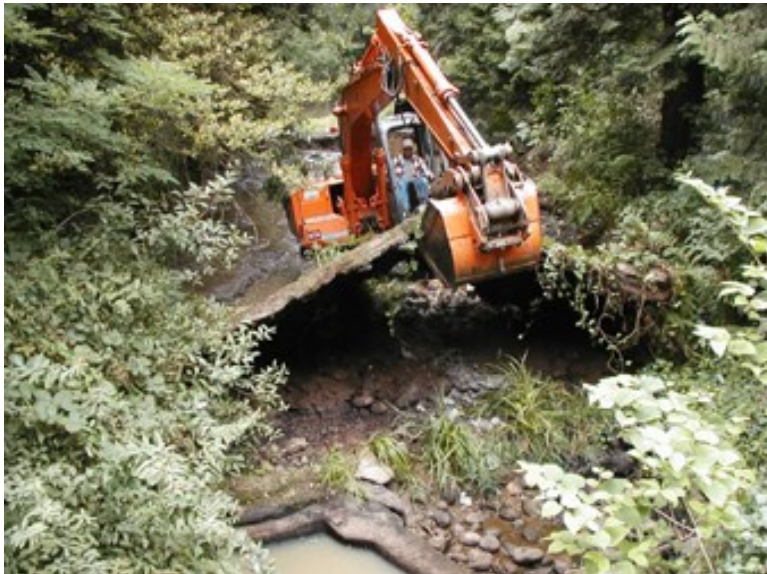
Figure 51. Removal of concrete weir in Johnson Creek, Portland, OR.
