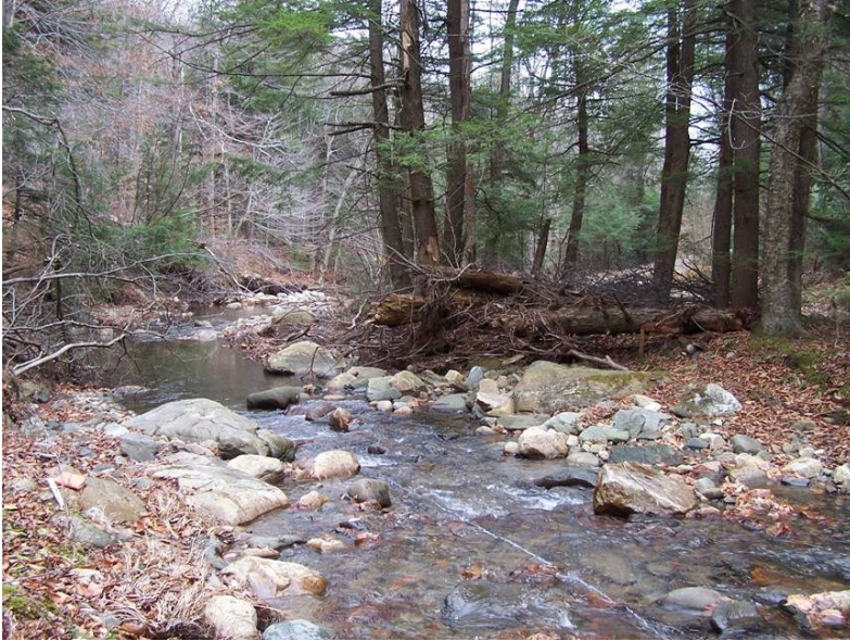
Figure 46. Series of rock steps installed for channel grade control, Tower Brook, Chesterfield, MA.
