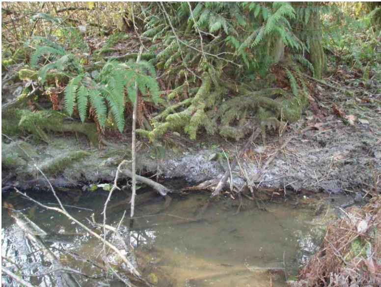
Figure 26. Photo of exposed root mass of Western Red Cedar (covered in moss) adjacent to Whipple Creek upstream of Union Road. Exposure of root mass suggests channel expansion (deepening) has occurred in this area.
