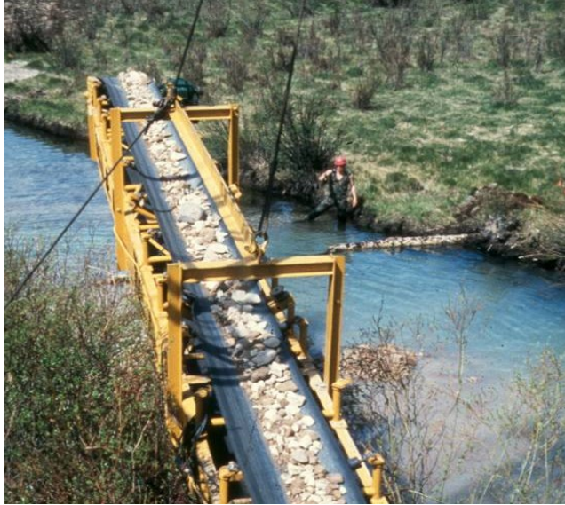
Figure 50. Conveyor placing substrate (cobbles and gravels), Ruby River, Montana.
