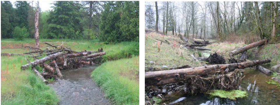
Figure 48. Large wood complexes installed for streambank protection (left, Kelley Creek, Portland, OR) and for habitat enhancement (right, side-channel of Clackamas River, OR).
