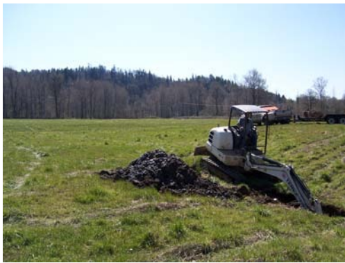
Figure D3. Test Pit 2 Excavation
