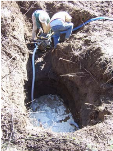
Figure D1. Test Pit 1 Excavation
