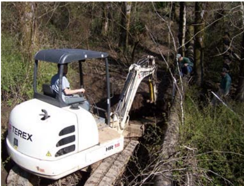
Figure D4. Test Pit 3 Excavation Area
