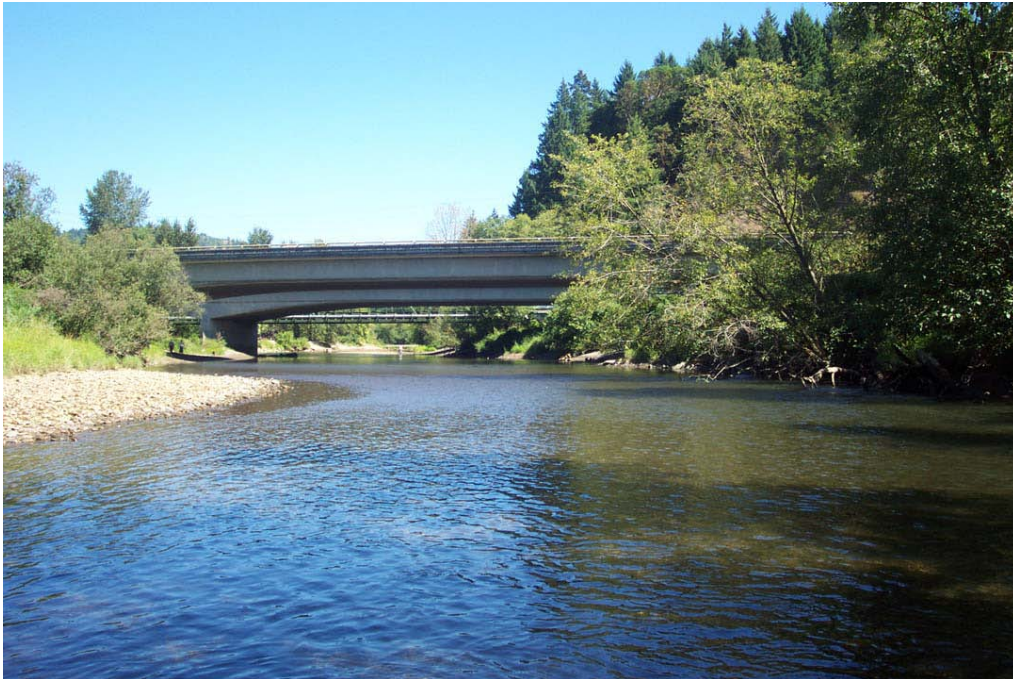
Photo 10 – Upstream view I5 Bridge.
