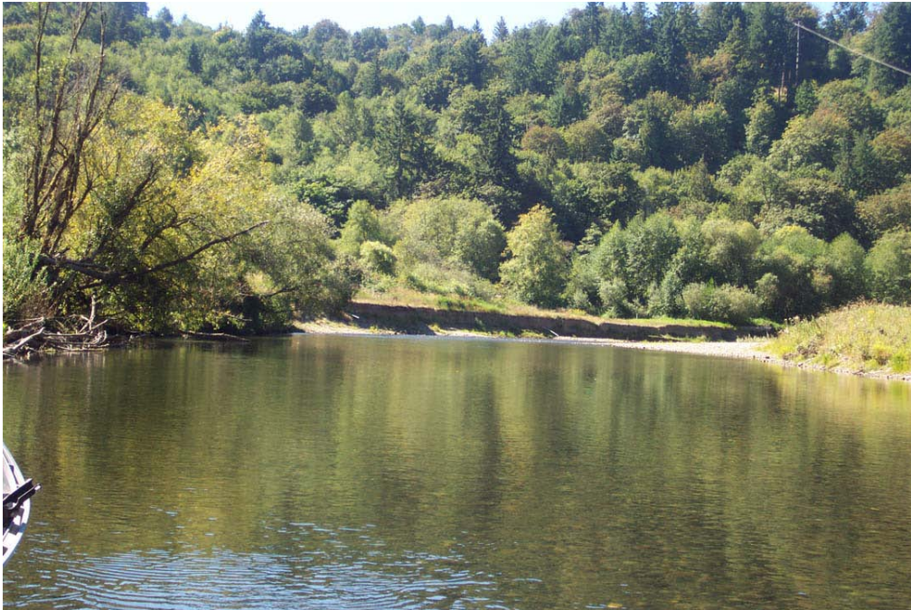
Photo 4 – View downstream of eroding bank on Ledgett’s property. Immediately to left is a small LWD cluster.
