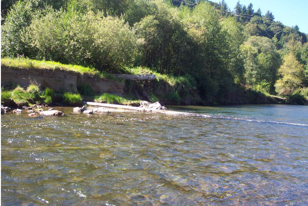
Photo 5 - Abandoned Gas line.
