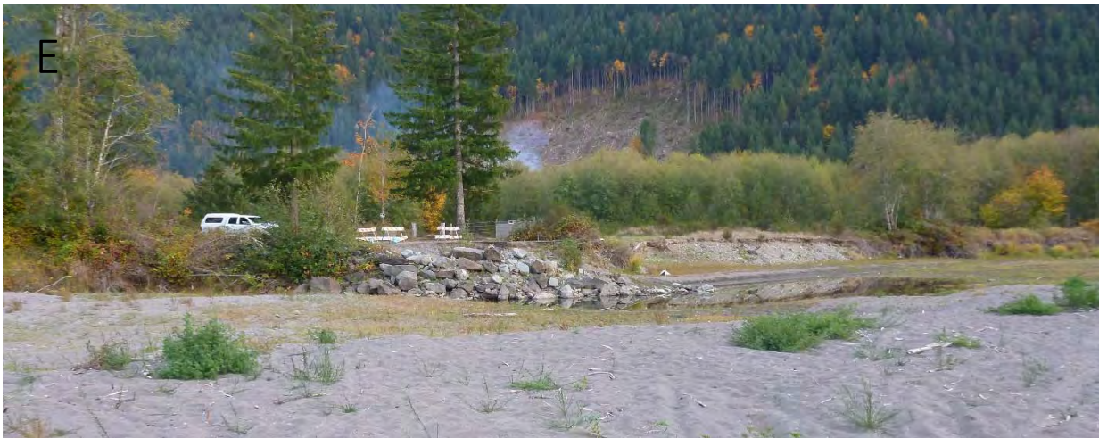
Figure 5. Representative images from the Cowlitz-Mid-Valley LU. A = riprap bank protecting houses river-right near RM. B = broad braid-plain typical of this reach (near RM 123). C = riprap failing into channel near RM 120. D = Elements of island-braided system downstream of RM 120. E = road washout (and now rock barb protection) river-left near RM 118.5.
