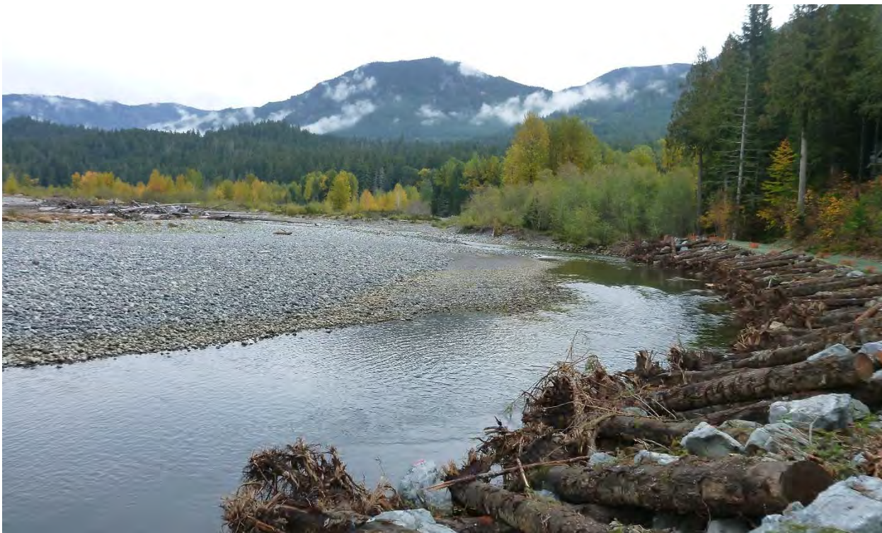
Figure 2. Recent bank stabilization project with large wood and riprap at RM 131.5 (Timberline community).
