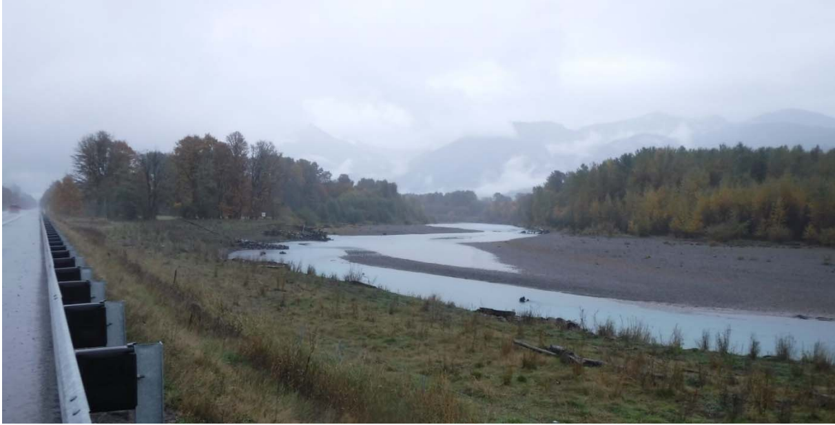
Figure 8. Bank stabilization adjacent to Highway 12 with barbs.
