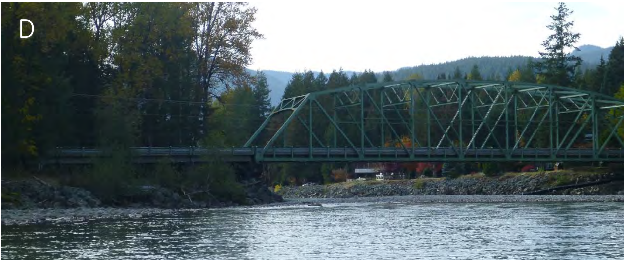
Figure 4. Representative images from the Cowlitz-Packwood LU. A = typical broad flat gravel and cobble bar. B = houses high on south bluff in Packwood area. C = Riprap and large wood bank protection structure on south bank upstream of Skate Creek Bridge. D = Skate Creek Bridge and riprap extending up- and downstream.
