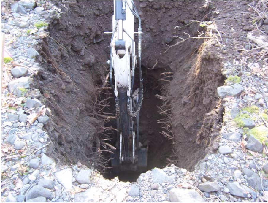
Figure 21. Excavation (typical) 8 to 10 Feet below Ground Surface.
