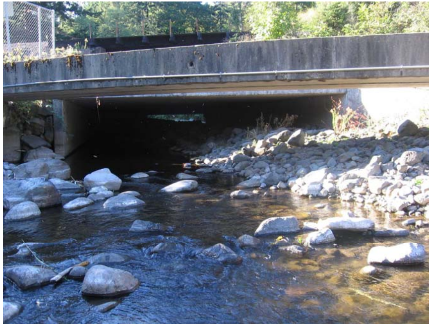
Photo 23 – View into Beacon Rock Moorage Road culvert from the downstream side
