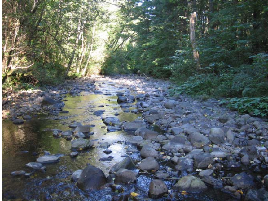
Photo 21 – Typical straight channel with uniform profile between Highway 14 and Beacon Rock Moorage Road culvert. Bed material is mostly large cobble and small boulder with some gravel and small cobble.
