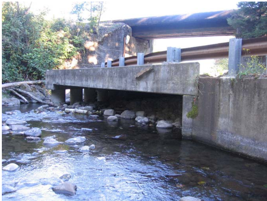
Photo 22 – Upstream side of Beacon Rock Moorage Road culvert crossing. Some bed load is depositing at the upstream end and possibly within the culvert.
