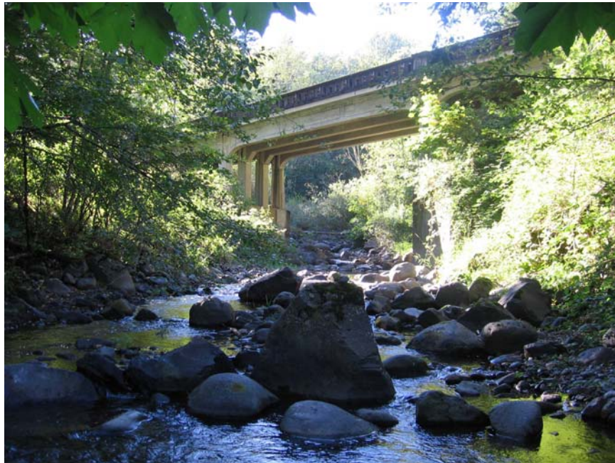
Photo 20 -- Looking upstream at Highway 14 Bridge
