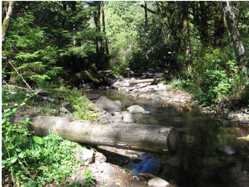
Photo 6 – Looking upstream at a series of alternating (left bank then right bank) log deflectors about 1,000 feet downstream of bridge, bed may have degraded and left structures perched.
