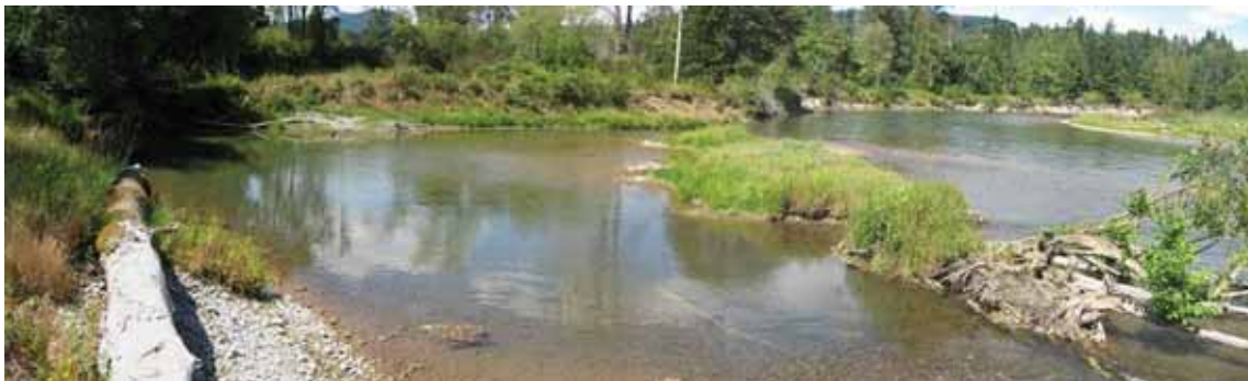
Figure 5. View of project site looking upstream
