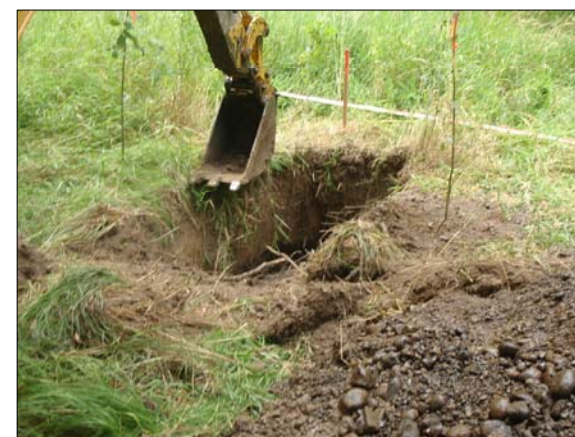
Excavation Area 6' x 6'
