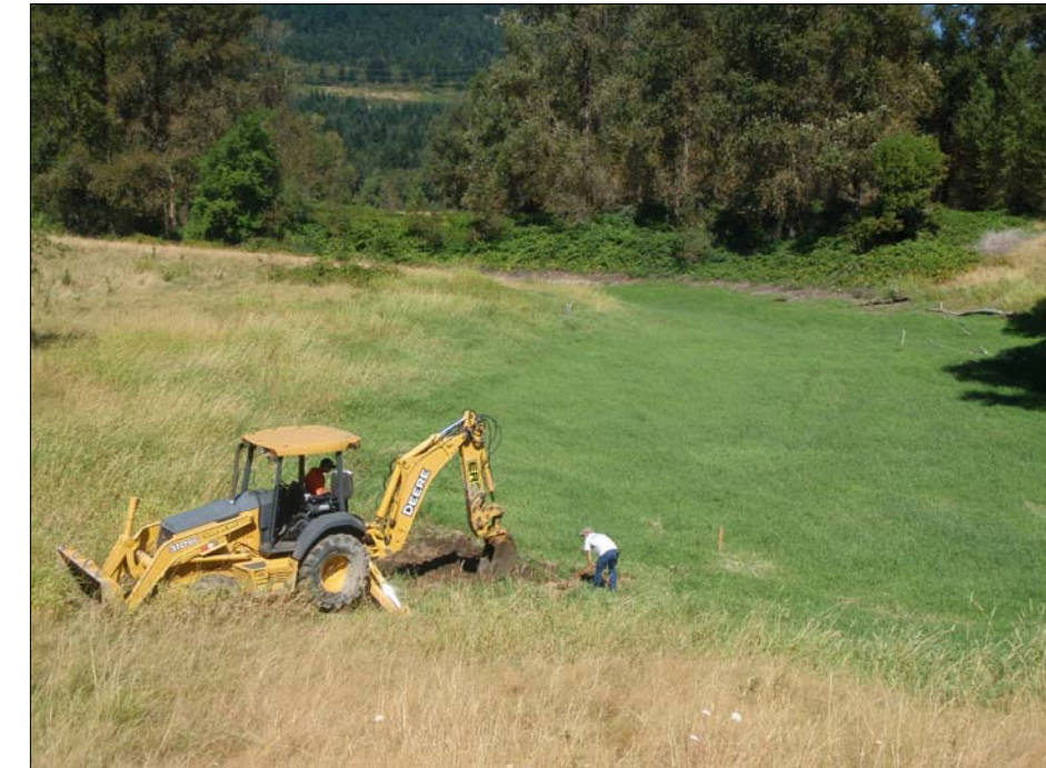
Typical Backhoe Staging For Test Pit Excavation
