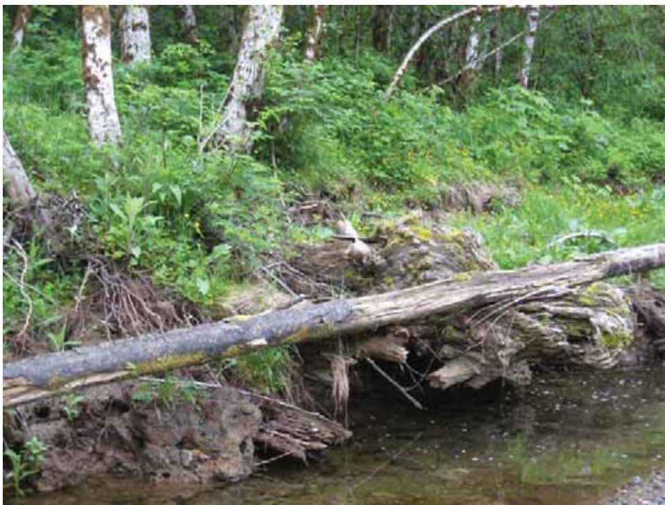
Figure 31. Buried Wood Exposed in Bank of West Fork Upstream of Hatchery Intake.
