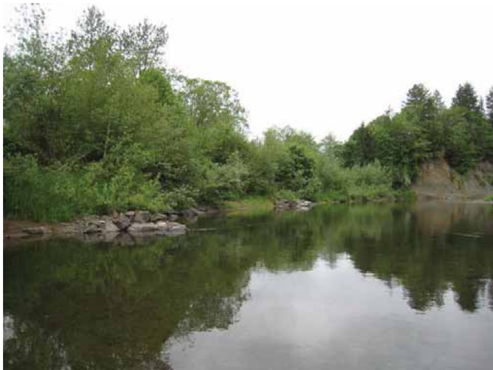
Figure 26. Groins and Vegetation along Left Bank in Reach 3.
