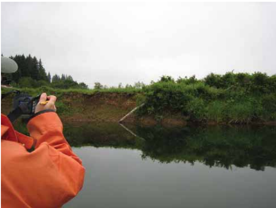
Figure 24. Eroding Bank with Limited Riparian Vegetation.
